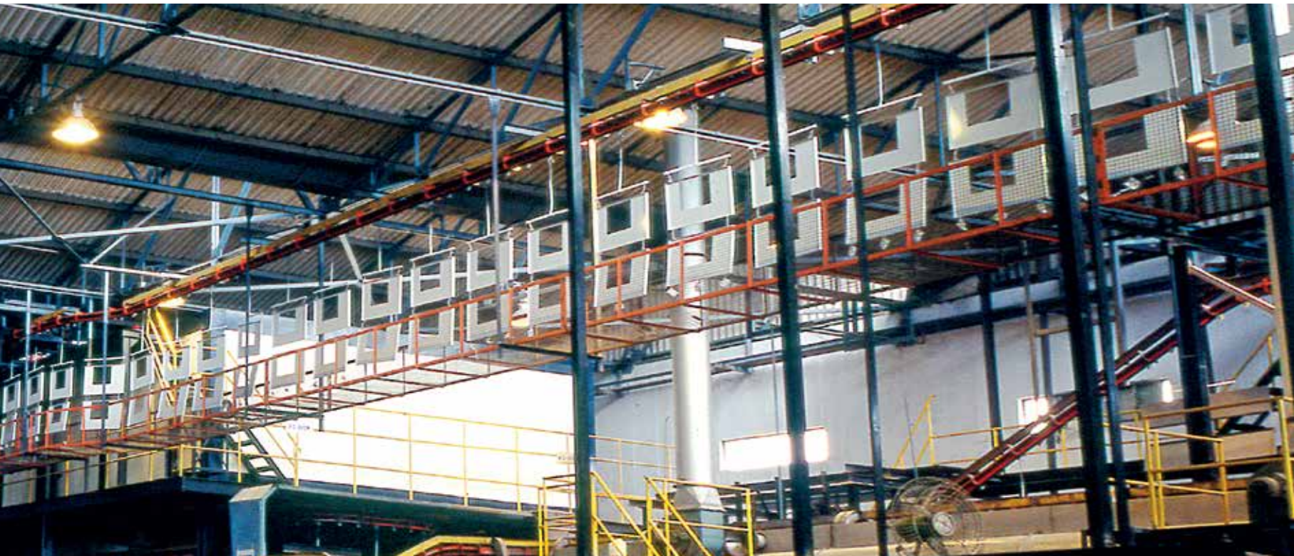
Paint shop at Dadra Plant
