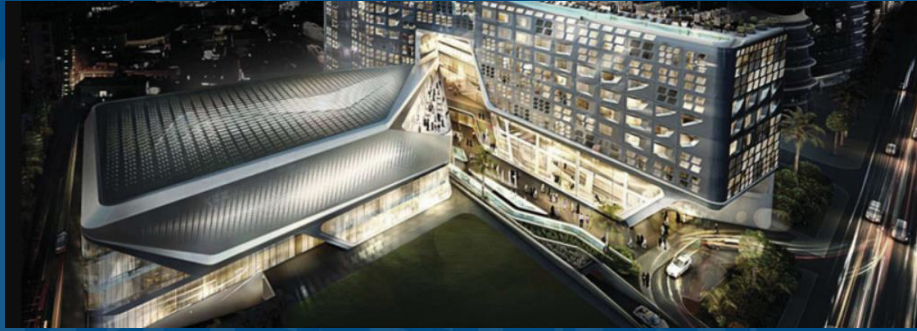
HVAC works in Doha Live, Qatar
