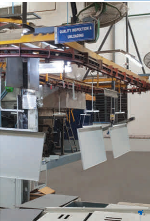
Powder Coating Plant at Blue Star's Wada manufacturing facility
