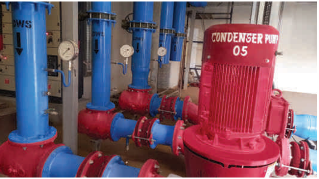
Condenser pump and piping work by Blue Star at TCS, Pune
