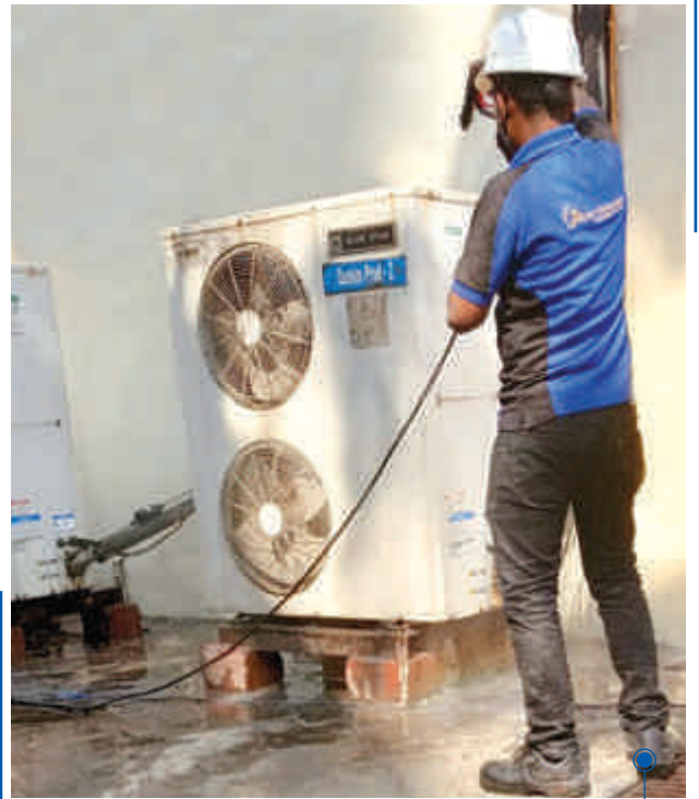
Blue Star's service technician cleaning an air conditioning outdoor unit
