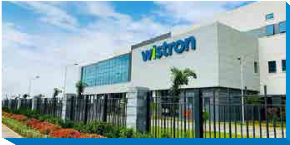
Mechanical, Electrical and Plumbing (MEP) works for Wistron Infocomm's factory expansion project, Bengaluru
