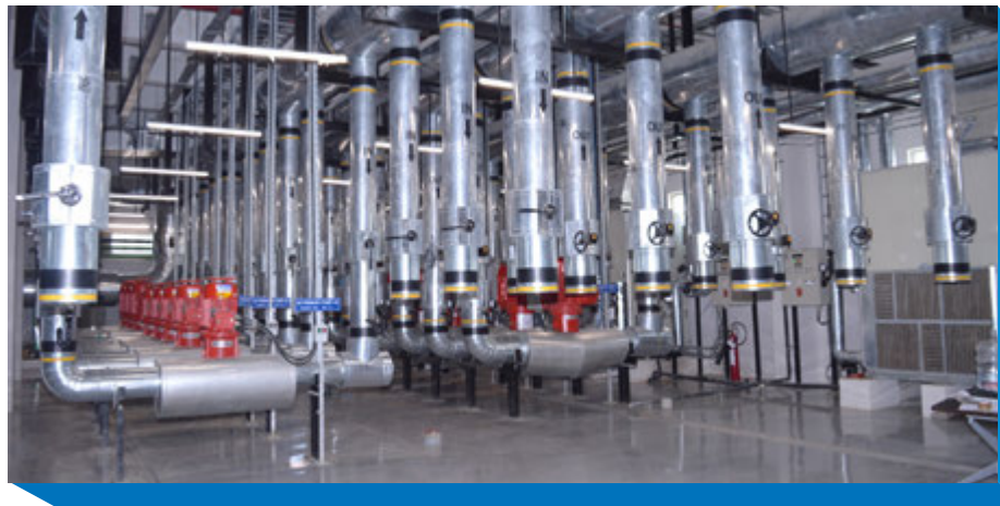
Chiller plant room installation at Ford, Chennai
