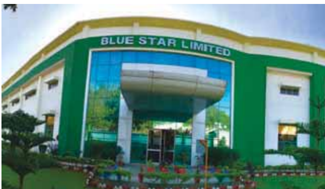
Blue Star's manufacturing facility at Himachal Pradesh
