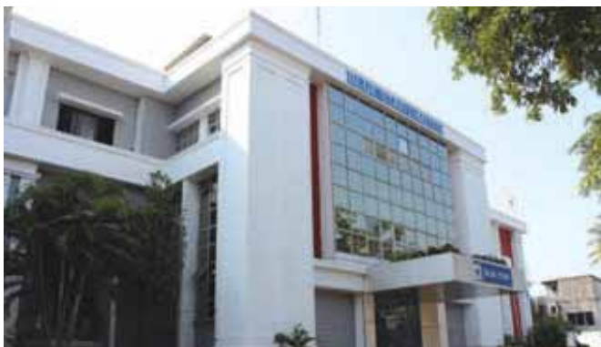
Blue Star's manufacturing facility at Dadra
