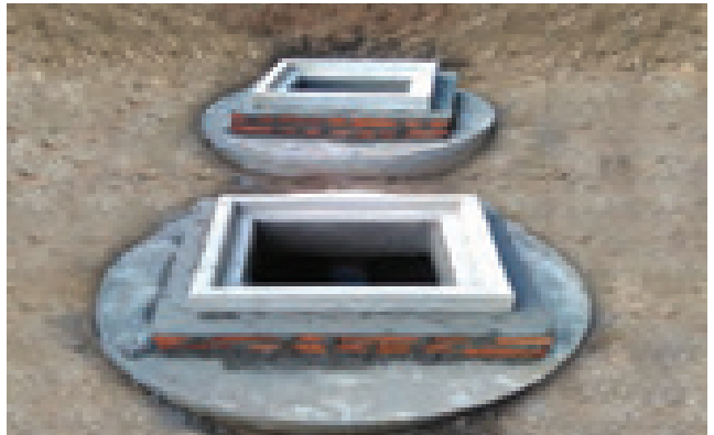
Recharge pits made for the rainwater harvesting plant at Dadra
