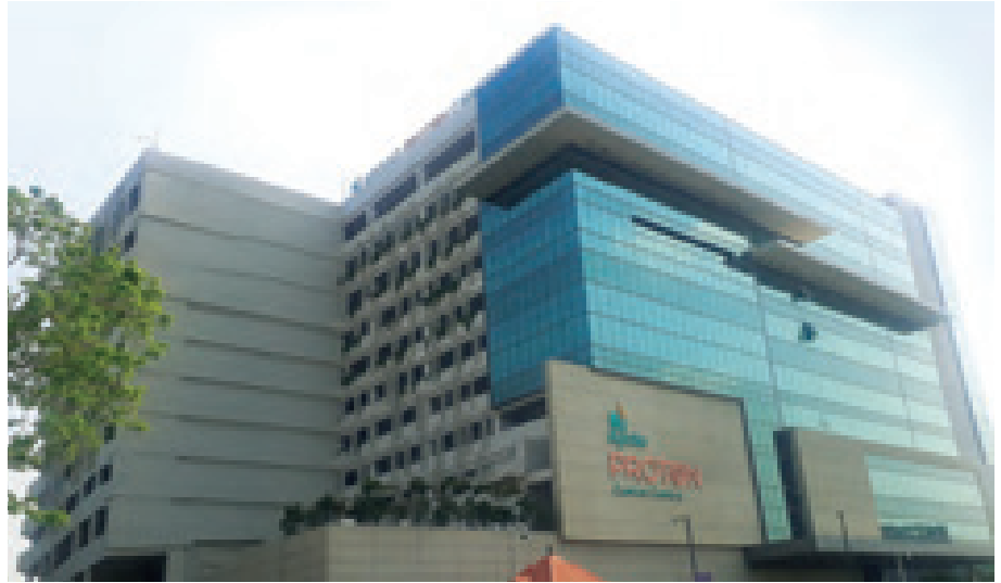
Integrated Mechanical, Electrical & Plumbing (MEP) services for Apollo Proton Cancer Centre, Chennai
