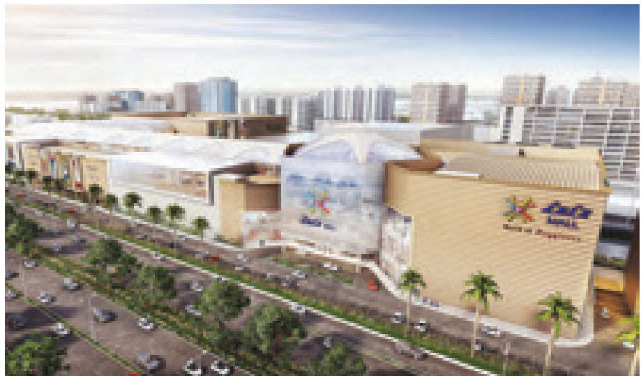
Integrated MEP (Mechanical, Electrical & Plumbing) services for Lulu Mall, Lucknow
