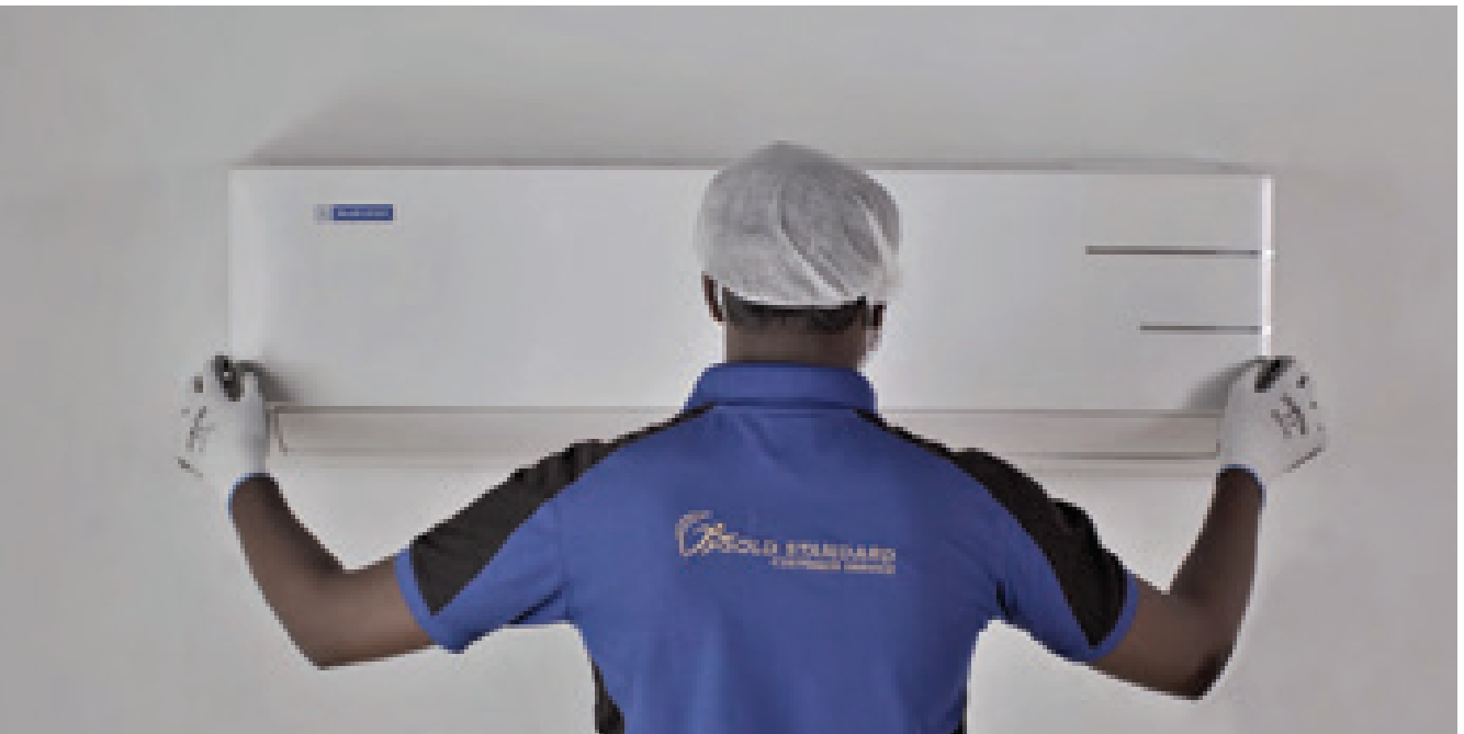
A split air conditioner being cleaned ensuring safety standards amidst the current pandemic
