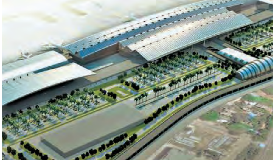
| HVAC services for Chennai International Airport
