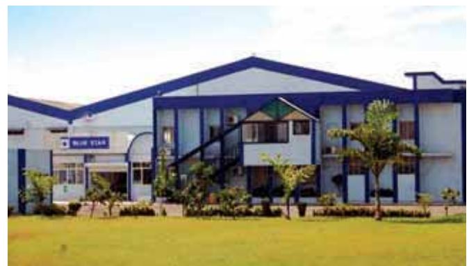
Blue Star's manufacturing facility at Ahmedabad
